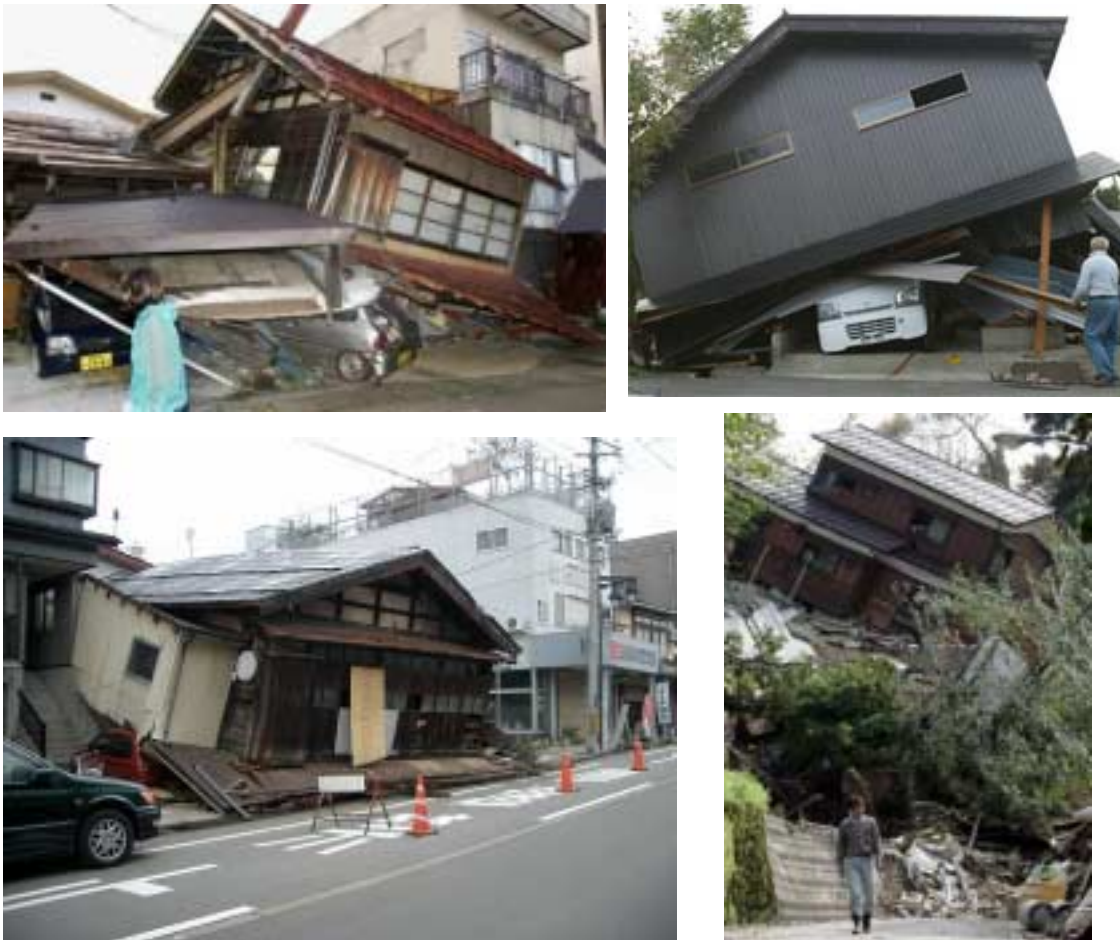
Figure 9.1: Collapse of wooden houses
