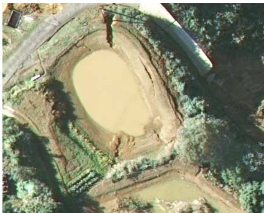
Figure 8.11: Embankment failures associated with earth dams
