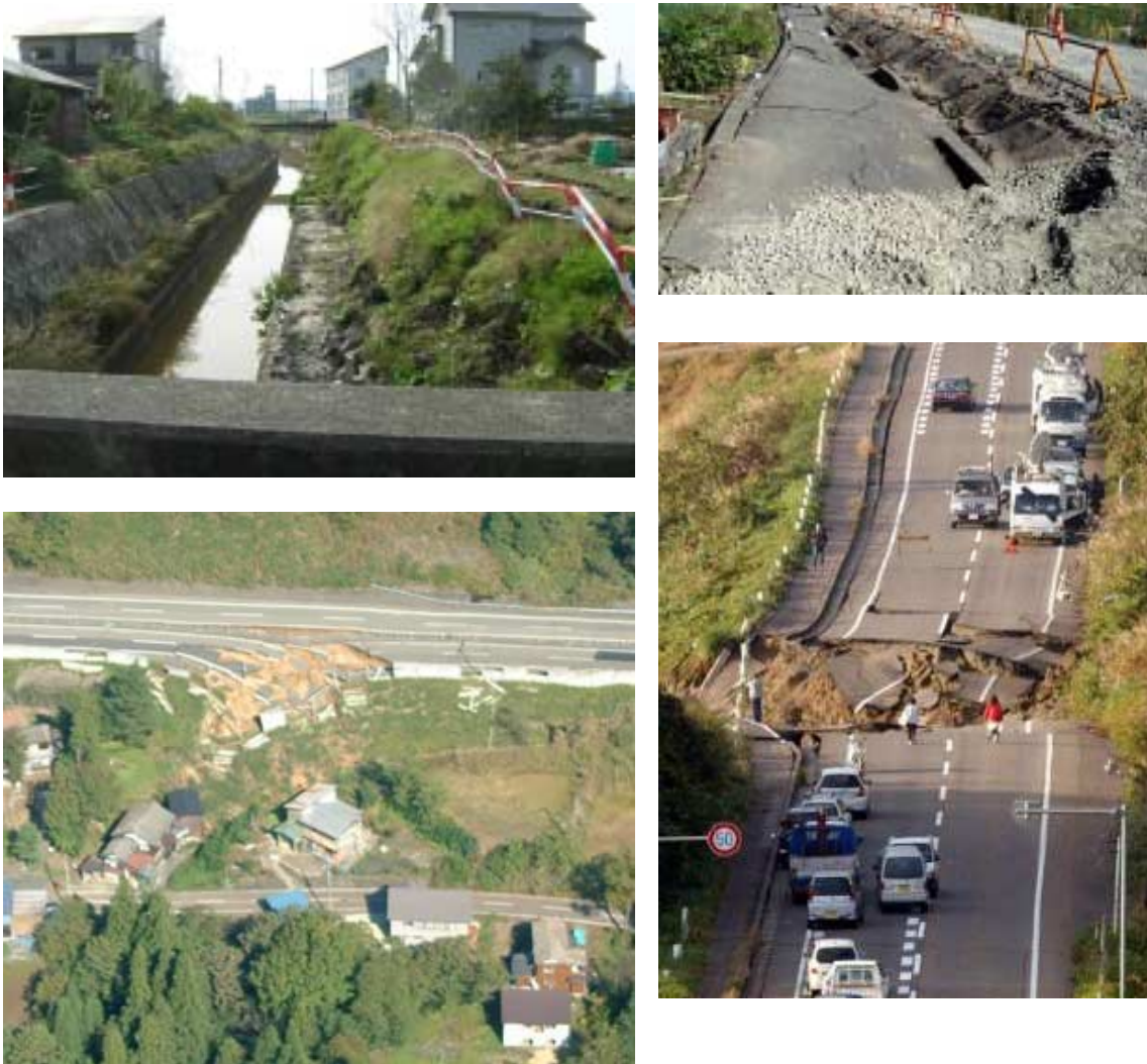
Figure 8.10: Embankment failures
