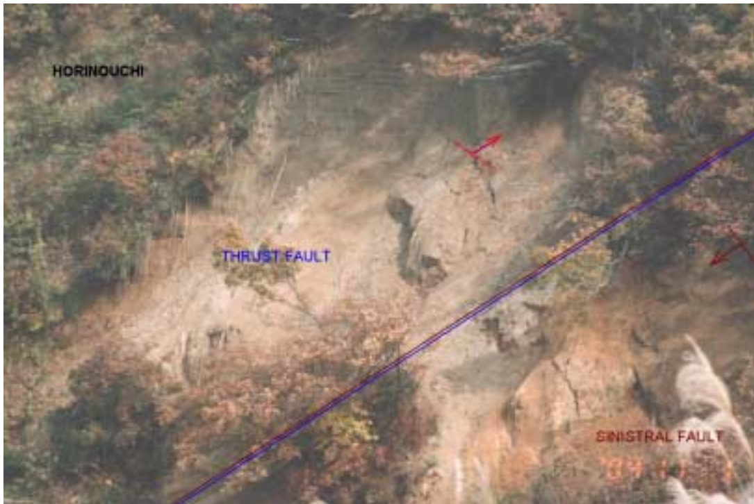
(b) Thrust and sinistral faults nearby Horinouchi along Kanetsu expressway
