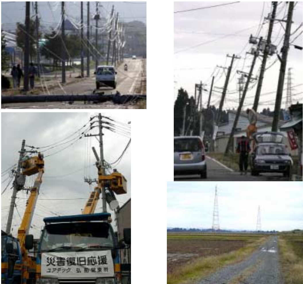
Figure 11.1: Damage to electric transmission lines (Pictures from various web-sites)
