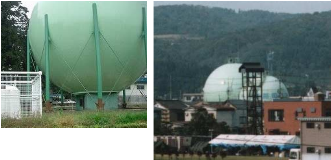
Figure 11.3: Non-damaged spherical gas tanks
