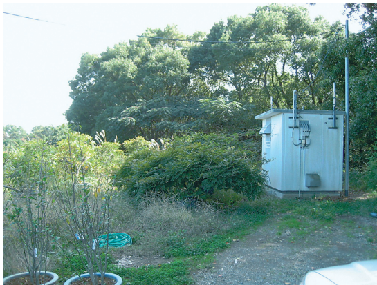
Fig. 20 A view of Shuzenji Station.
