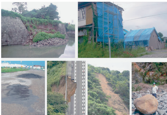
Fig. 7 Views of some damage caused by the Suruga Bay earthquake.
